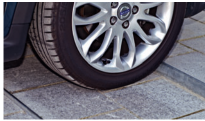
04 E The tire position for the upper parking place with a fixation integrated into the stone paving is effective and well-designed.
